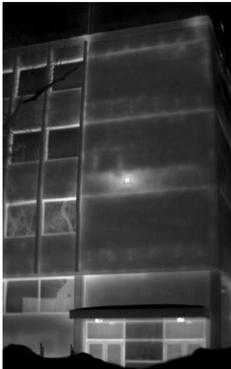
Figure 8. Negative Building Pressure (-140 Pa), T_o = -11^\circ\text{C}
