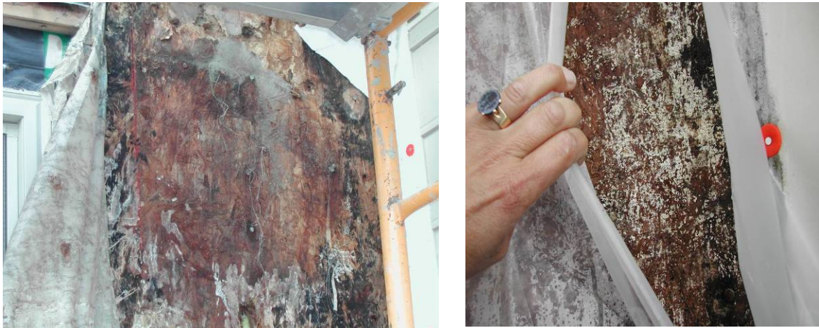
Figure 6. Destructive testing is necessary to confirm what IR has indicated
